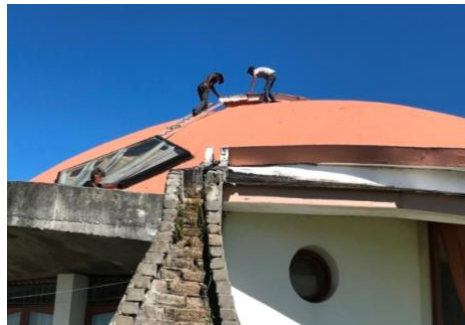
Henry & Garikayi - Fixing the roof
